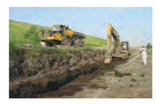
HIS Constructors, Inc. (HIS) was contracted by the Illinois Environmental Protection Agency (IEPA) to import and place structural fill and clay for the construction of a cap on the Paxton landfill.
