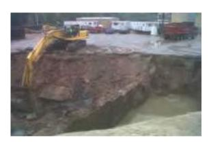
HIS Constructors, Inc. (HIS) was contracted to perform the excavation, transportation and disposal of 20,000 tons of MGP impacted soil and debris.
