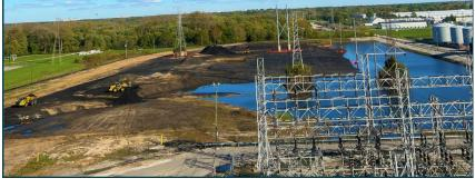
The generation station had ceased burning coal and removed the usable coal from the site. However, residual coal and coal fines remained that were required to be removed prior to regrading the coal yard area.
