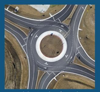
In addition to the utilities, HIS constructed the new roundabout and performed almost all major activities except the paving. Traffic management for the surrounding business was a primary concern as the road had to stay open to accommodate trucks. The road was built on a 4" subbase of cement stabilized soil.
