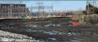
The original plan had the excavation of 130,000 CY residual coal fines and transporting excavated material to landfill. We presented an alternate beneficial reuse approach that recycled a large percentage of coal product and saved significant costs. This approved reclamation approach resulted in 260,000 tons of material diverted from landfill disposal.
